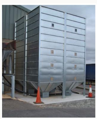
A 50.0 ton capacity pellet store measuring 4m x 4m x 6m high was first assembled on site and then a dual auger system transporting the pellets from the silo to a bucket elevator was installed.
