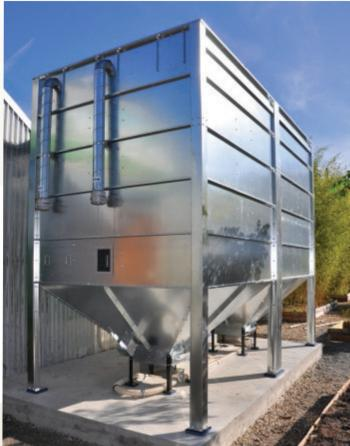
Pellets are pneumatically fed into the boilers and hot air is then blown through textile ducting into the growing area. The blow heaters are connected to a sensor control system in order to keep the greenhouse at the exact temperature required all year round.
